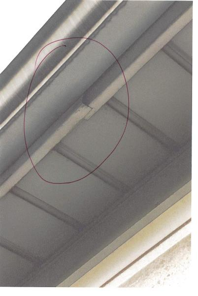
the Circled red is damage under neath the gutter on the front of house to soffit and fasia/Aashing is damaged
