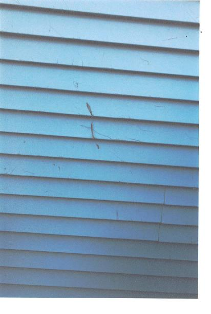
\* This is more damage to the siding on the upper front side of the house (facing from the Street)
