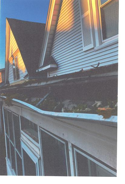
\* Pictured here you can see gutter damage along with flashing damage and Shingle damage
