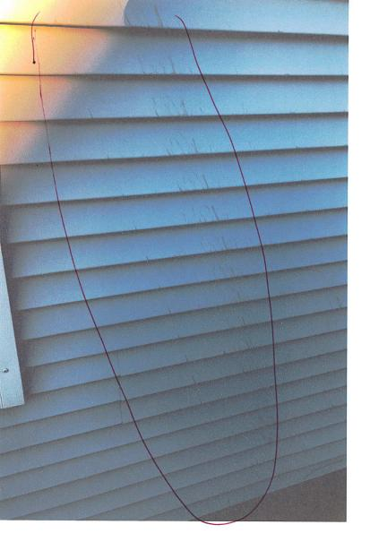
\*Circled in red the Siding is damaged
