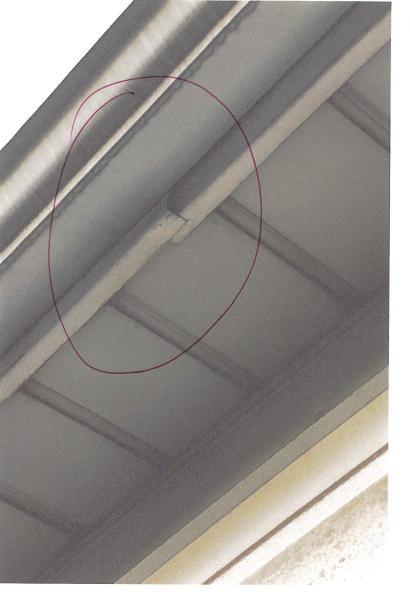
\* Circled red is damage under neath the gutter on the front of house \* soffit and fasia/Aashing is damaged
