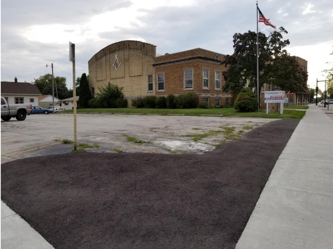
Staff recommends that the parking lot be repaved in order to provide a more aesthetically pleasing lot without cracks and loose pavement. Additionally, staff recommends replacing the wheel stops with a curb, in order to better delineate the landscaped area between the parking lot and sidewalk. Staff also recommends adding trees or shrubs in the landscaped area between the parking lot and sidewalk.
