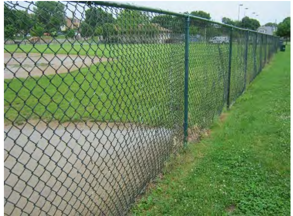
Fence is bowed from balls being hit into it
