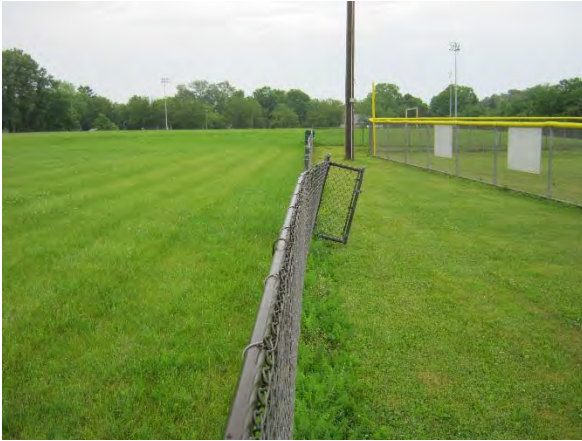
Soccer field fence in poor condition/bent in some areas
