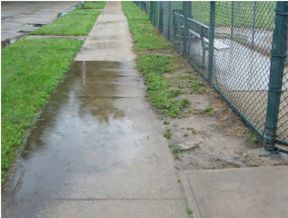
Erosion from northwest ball field onto sidewalk
