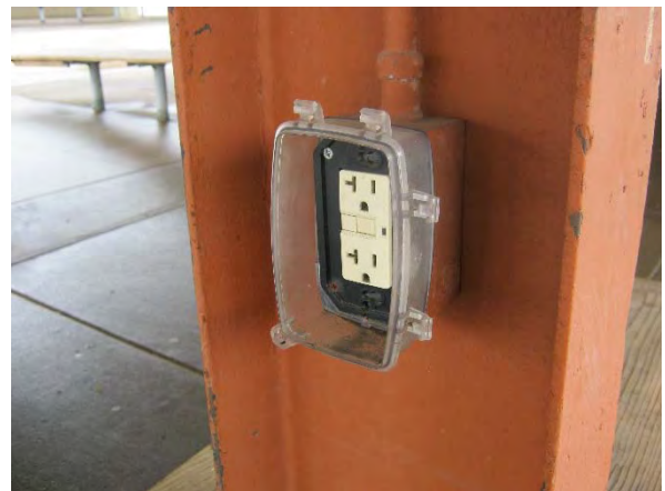
Missing electrical outlet cover
