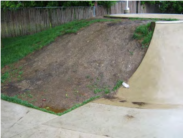
Erosion at slope on north side of park
