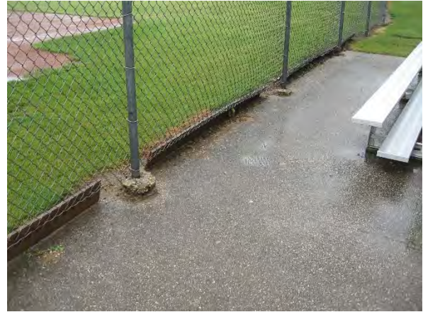
Gap at bottom of fence on 1 st base side
