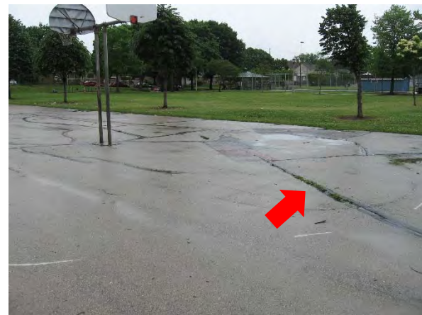
Weeds growing through cracks in court
