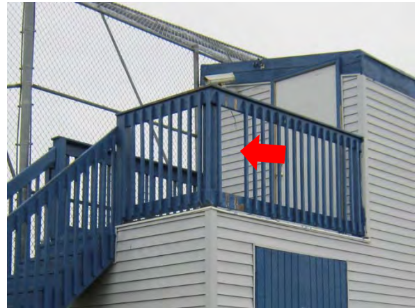
Missing boards on press box deck
