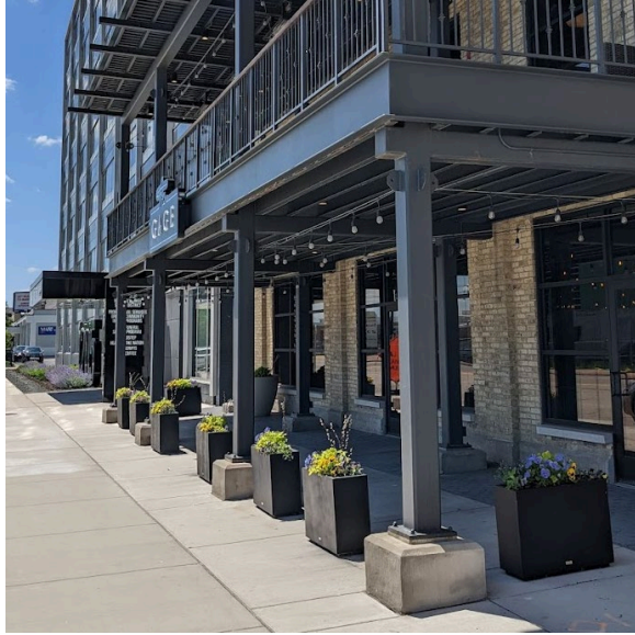
iv. This balcony addition references the historic industrial feel of the building while playing on the complementary colors of a neighboring building.
