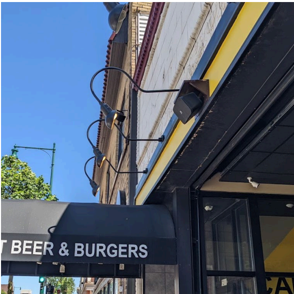
iii. Shielding lighting from public view highlights building features and signage while limiting glare to the sidewalk and neighbors.
