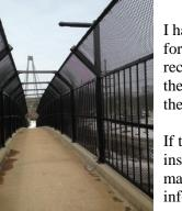
I have attached pictures of a recently completed lighting and fencing system for your reference that was used on a pedestrian structure over US 45 recently. These pictures depict a similar installation to what would be used at the Dakota Street Bridge. The LED lights would be built monolithically with the fencing on the structure.
