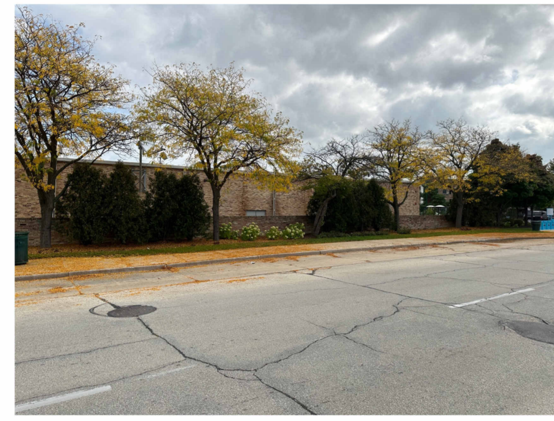
EXISTING LANDSCAPING AT WEST FACADE 9/29/23
