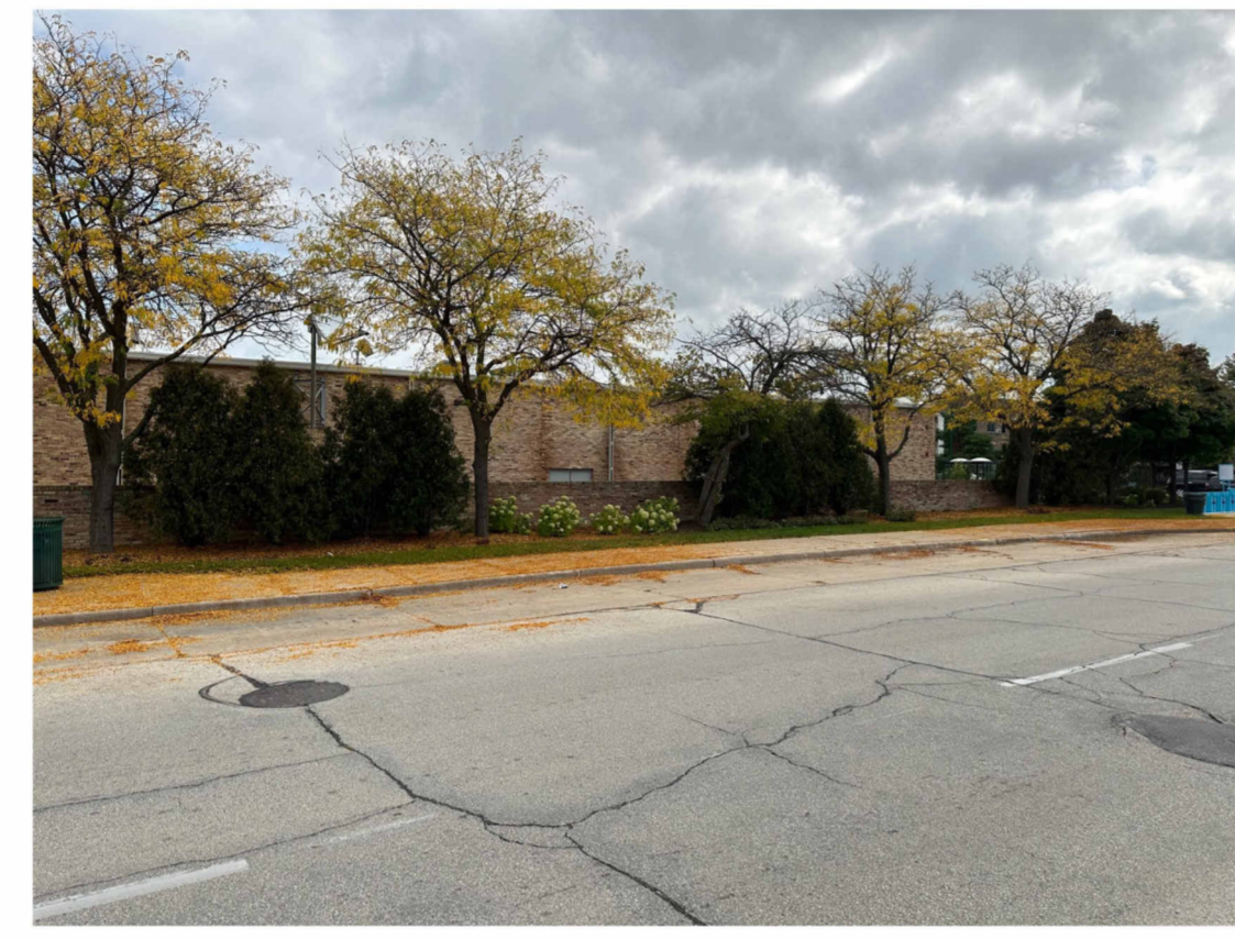
EXISTING LANDSCAPING AT WEST FACADE 9/29/23
