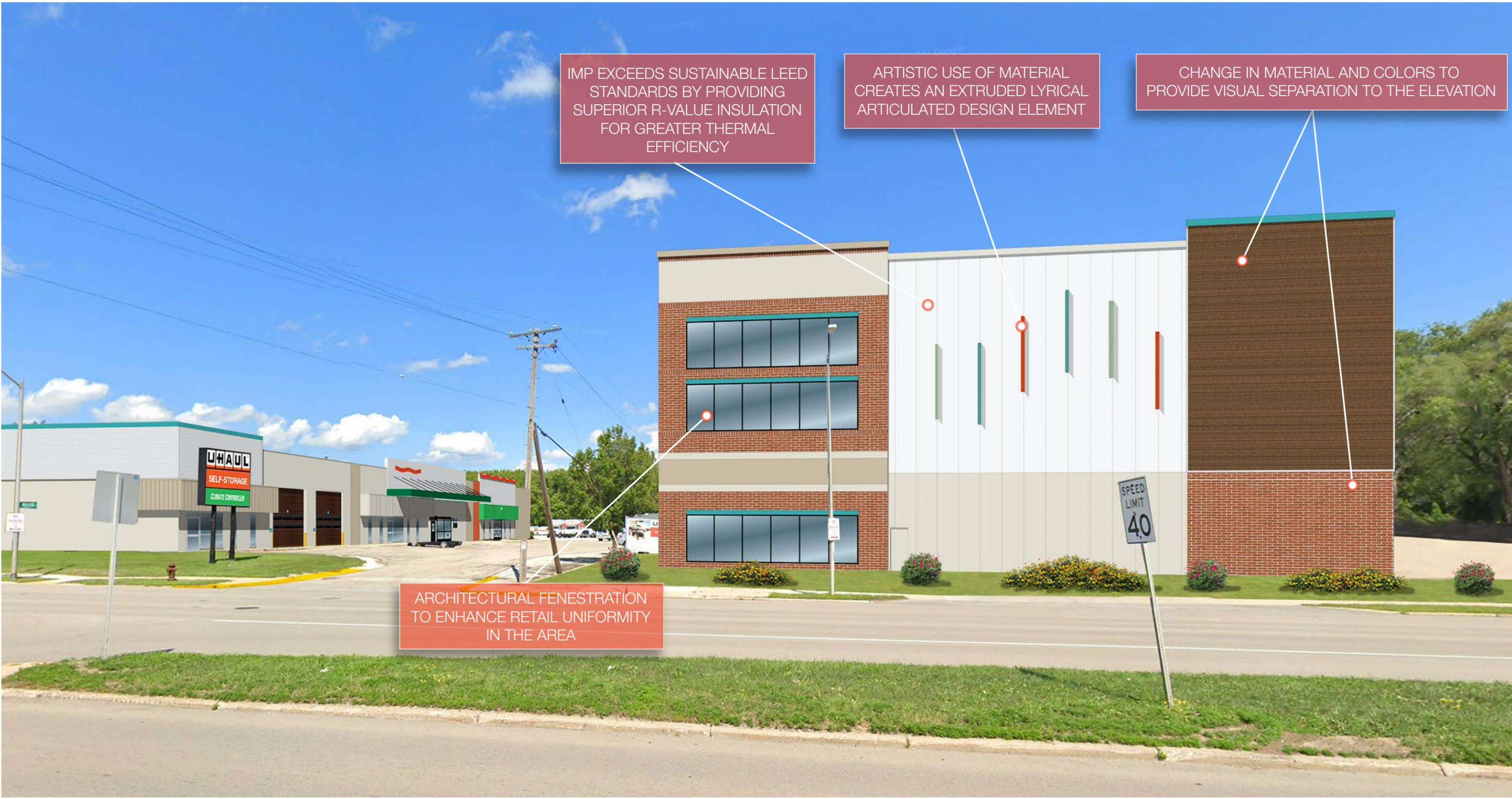
IMP EXCEEDS SUSTAINABLE LEED STANDARDS BY PROVIDING SUPERIOR R-VALUE INSULATION FOR GREATER THERMAL EFFICIENCY
