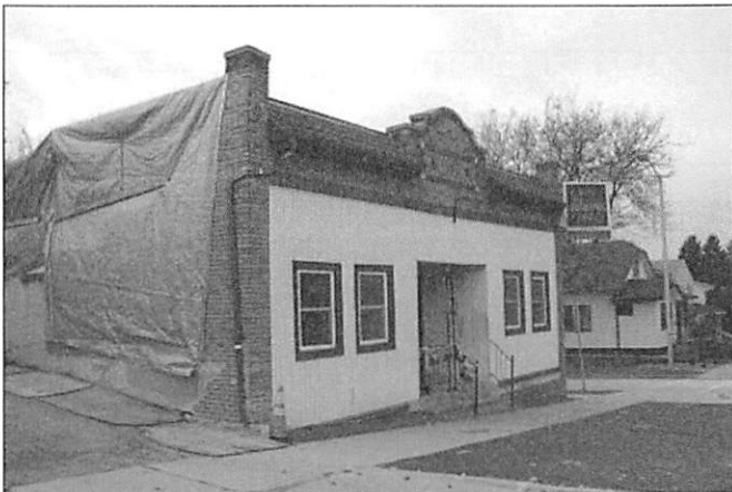
VIEW FROM NORTH EAST
