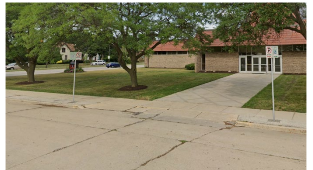
Existing curb cut that is recommended to be removed
