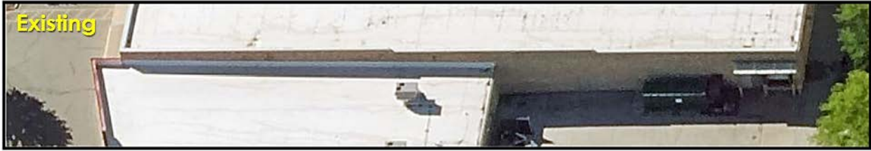
EXISTING NORTH EXTERIOR STOREFRONT
