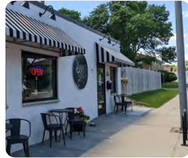
i. Orienting towards the street frontage enables an active streetscape and sense of place.
