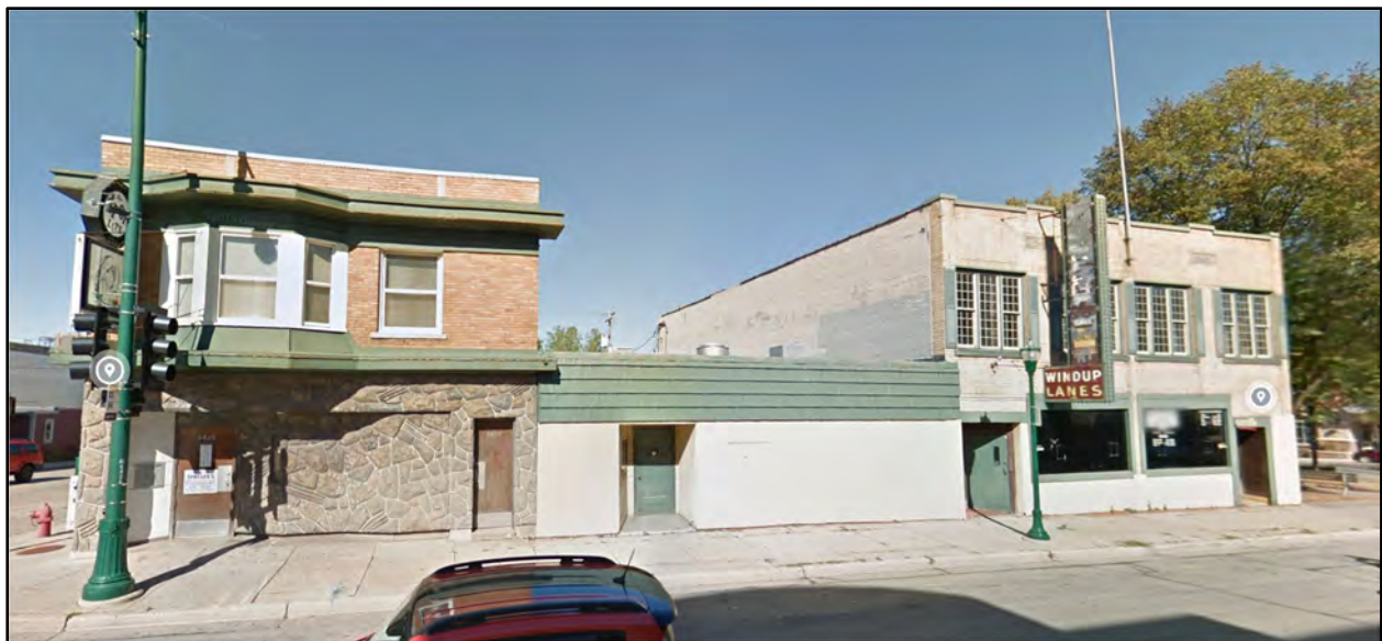
Google Street View of Existing Structures located at 6416, 6422, 6424 and 6426 W. Greenfield Avenue
