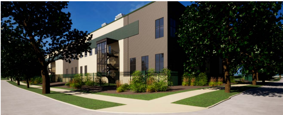
Views: Looking SW from the corner of S. 89 th and Mitchell St.
