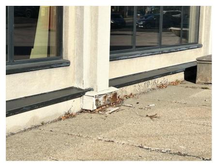
Generally, the building's façade appears to be in good condition. However, there are some sections of the façade that area crumbling and require repair, though those areas are few in number. Staff recommend the removal and replacement of any existing stucco façade features in disrepair, such as the region pictured to the left:
