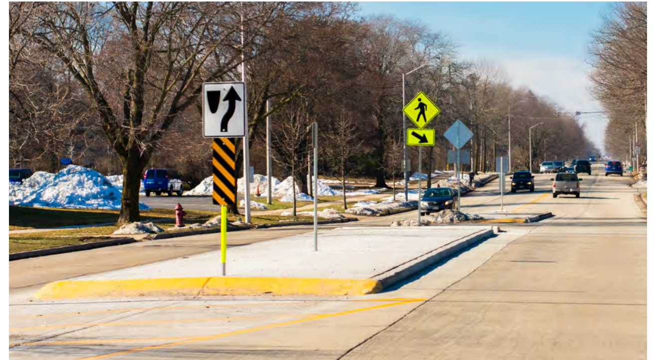
Newly constructed median and crosswalk at W. Lincoln Ave. & S. 117 th St. near West Allis Nathan Hale
