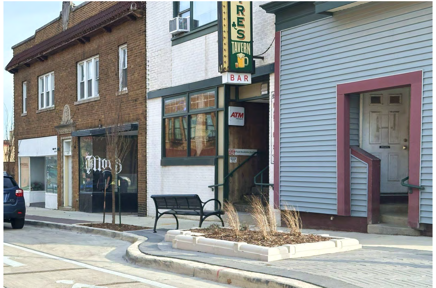
Bike lane, bump-out, green infrastructure, and public seating at W. National Ave & S. 63 rd St.
