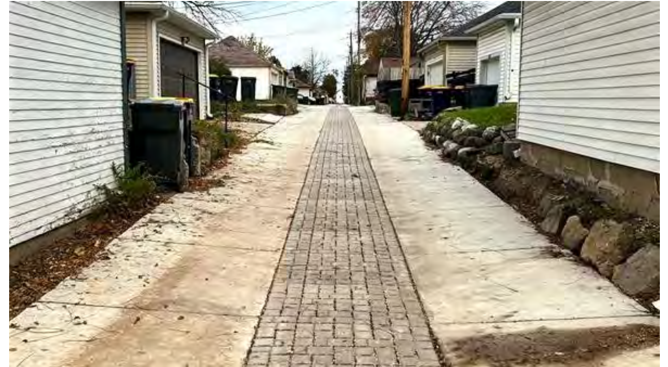
Alley reconstructed with permeable pavers to allow for capture of stormwater
