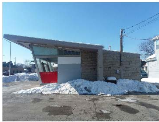
PHOTO OF EXISTING EAST ELEVATION
