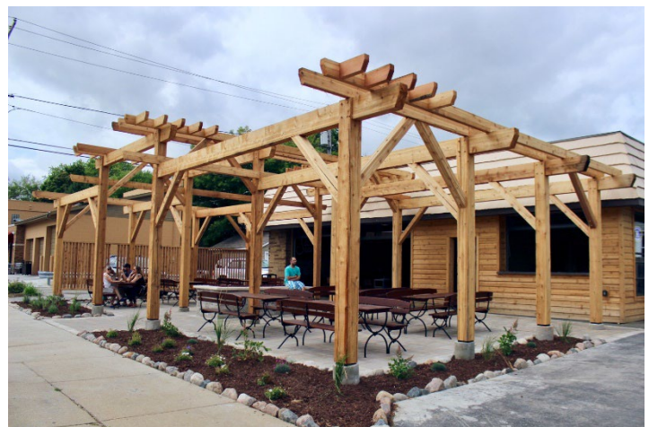
Station No. 6 Outdoor Patio (former parking area)
