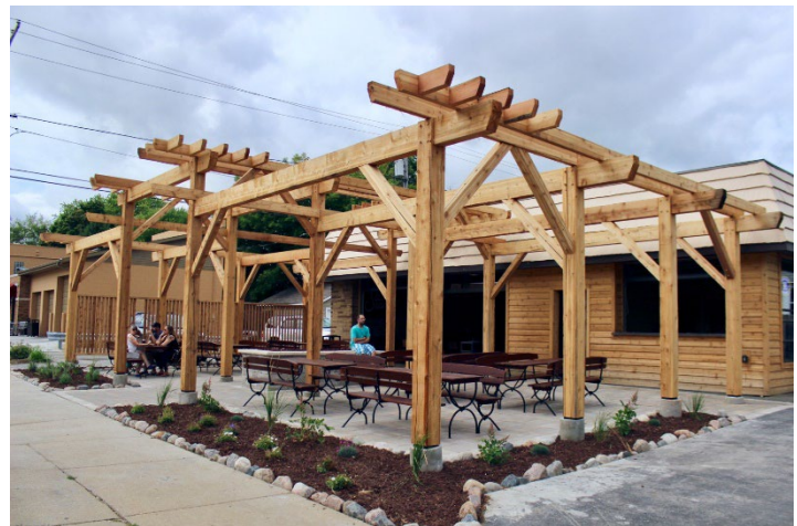
Station No. 6 Outdoor Patio (former parking area)
