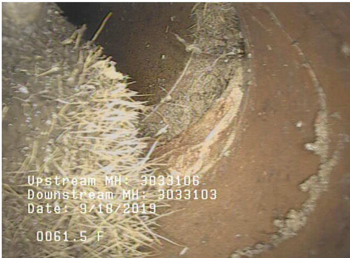
Photos of connection at city sanitary sewer main
