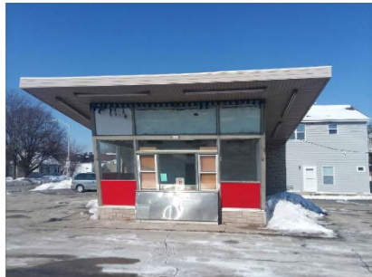
PHOTO OF EXISTING SOUTH ELEVATION
