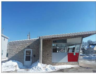
PHOTO OF EXISTING WEST ELEVATION
