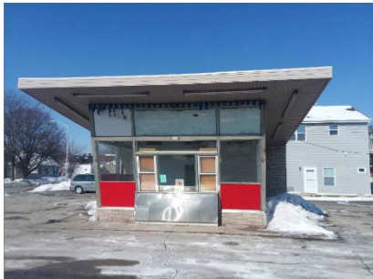
PHOTO OF EXISTING SOUTH ELEVATION
