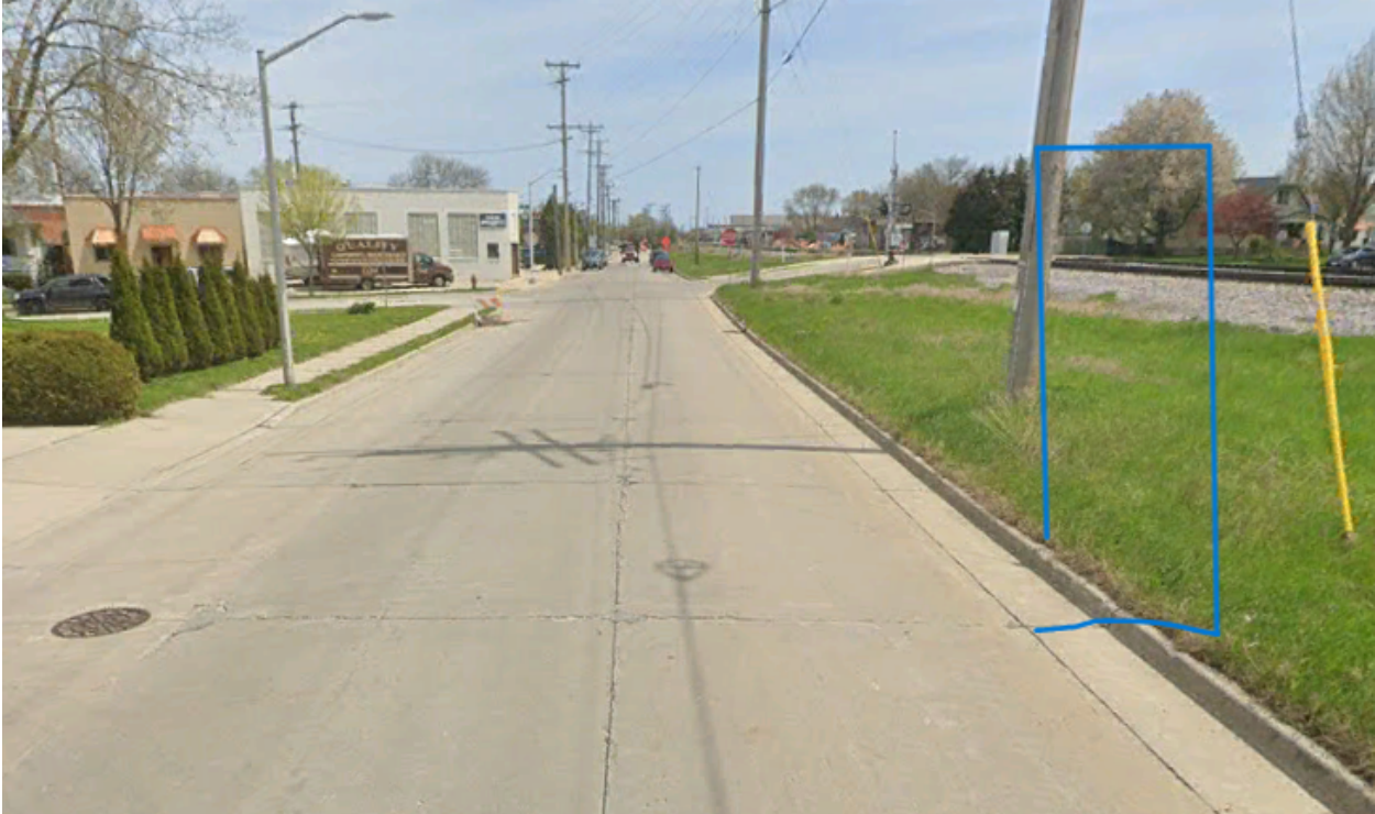
Parallel AWS missing from the eastbound lane of the northern W. Mobile Street
