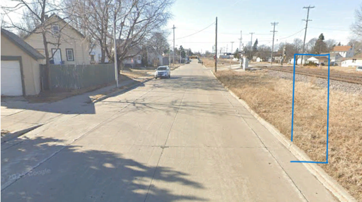
The parallel AWS is missing from the westbound lane of the southern W. Mobile Street
