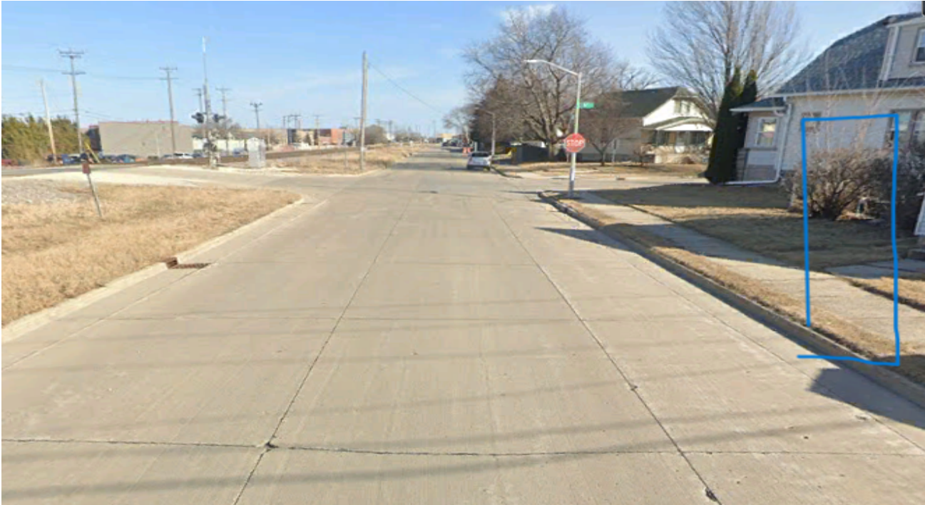
Parallel AWS missing from the eastbound lane of the southern W. Mobile Street
