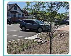
ii. Grading and draining impervious surfaces to bioswales and rain gardens filled with native plantings absorbs stormwater at the source, preventing runoff, pollution, and flooding downstream.
