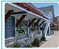
iii. Integrating awnings, stairwells, and other exterior features into the design adds depth and leads to a more coherent and pleasing appearance.
