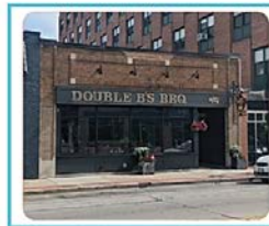
iv. An organized facade, large and proportional windows, and a strong palette of materials and textures forms the basis for a harmonious design that is attractive and functional.
