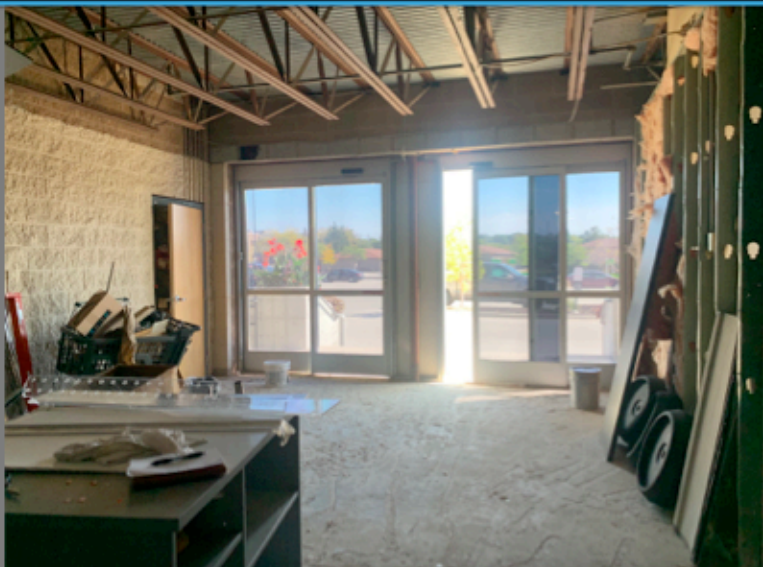
VIEW OF ENTRANCE FROM INSIDE
