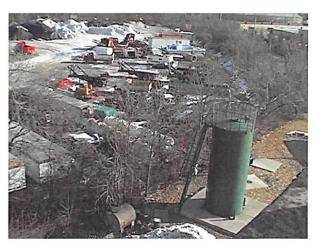
for placing footings & foundations will have to be removed from the site. The additional handling, trucking and disposal costs will be considerable. Any remaining suitable fill will still have to be compacted in about 8" to 12" lifts.
