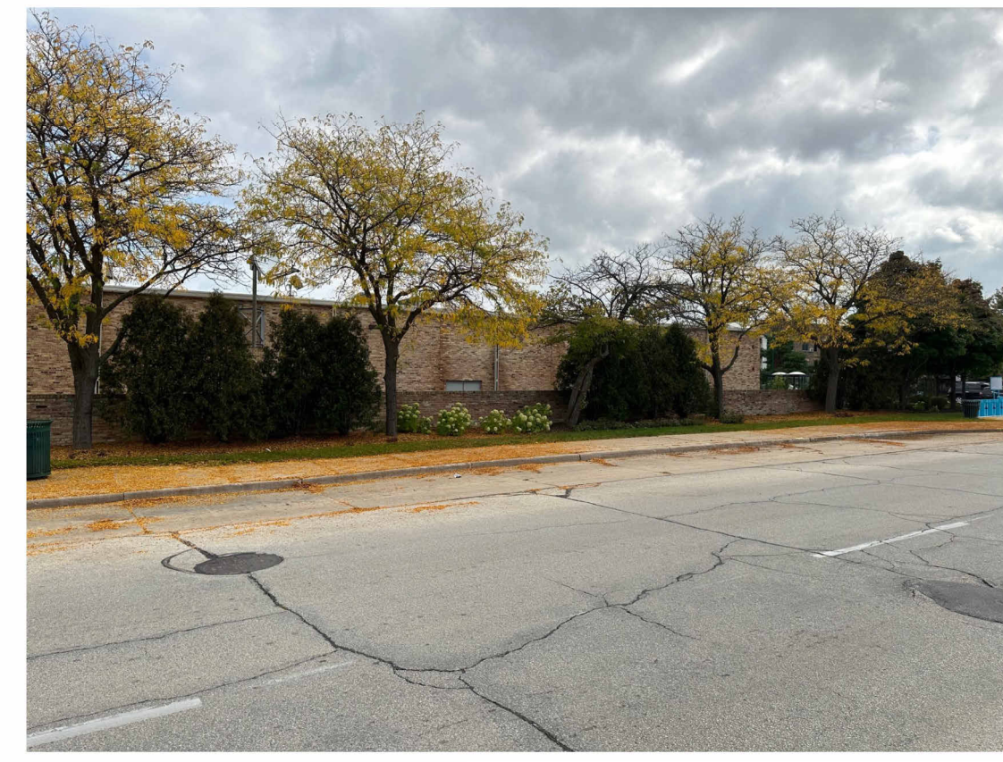
EXISTING LANDSCAPING AT WEST FACADE 9/29/23
