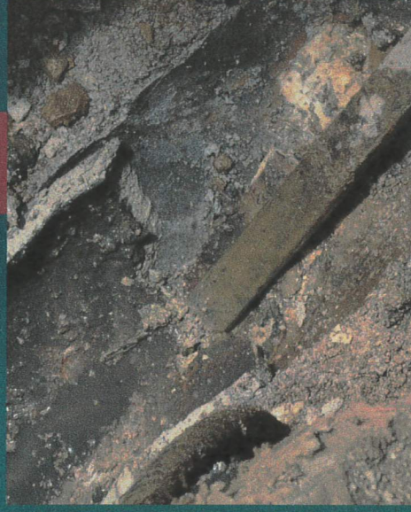
Concrete Under Lateral
