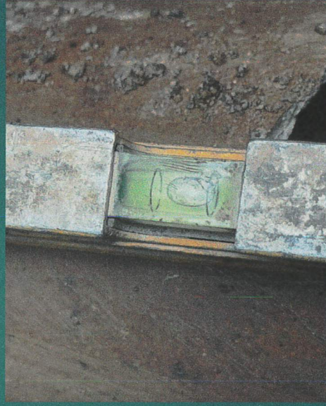
Back Pitch on Pipe (level)
