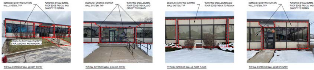
6E DEMOLITION PICTURES - FIRST FLOOR
