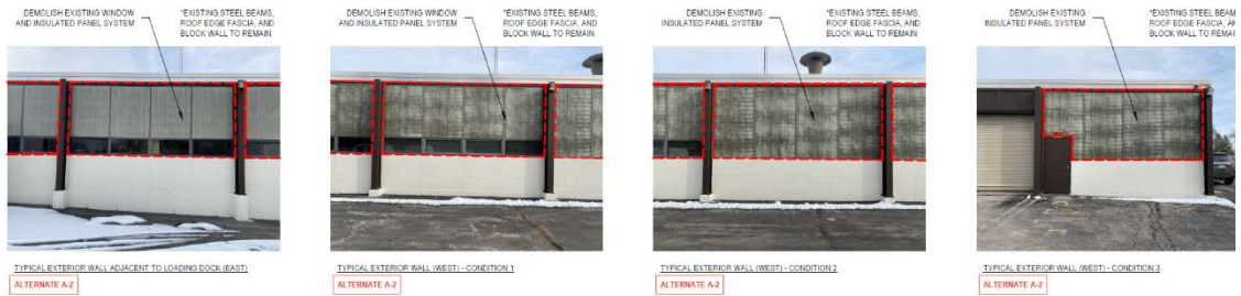
6E DEMOLITION PICTURES - LOWER LEVEL / ROOF
