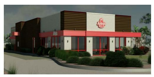
All four facades of the building will be updated with a more modern look. For the northern (front) half of the building, the existing metal coping, lighting, and red canopies will be removed. Thin brick (white & sable) and LP Smartsiding (brown) will be added on top of the existing masonry. Updated lighting fixtures and new metal canopies (red) will also be added.
