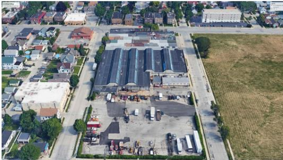
OVERALL EXISTING SITE CONDITION VIEW NORTH
