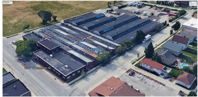
OVERALL EXISTING SITE CONDITION VIEW EAST
