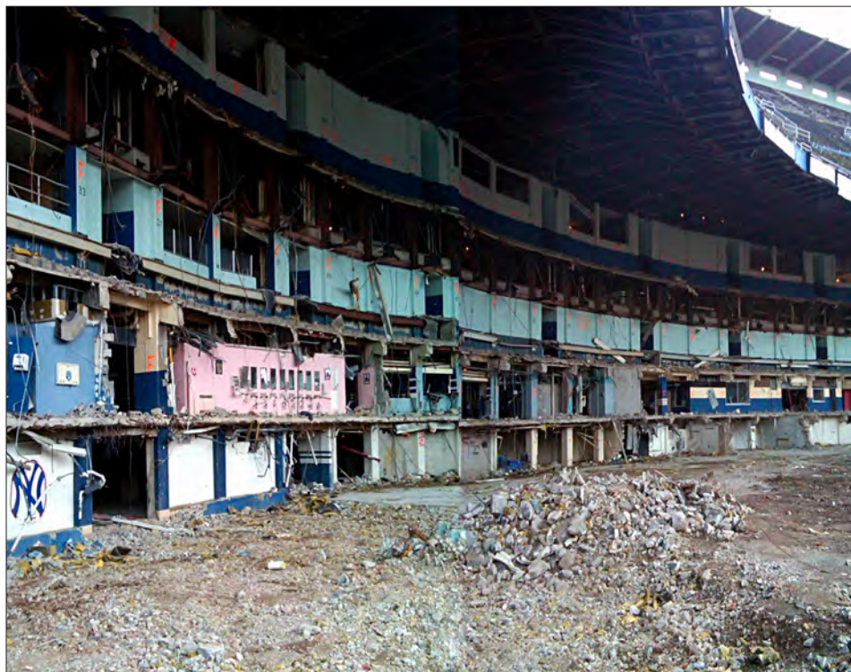
Hazardous materials and demolition assessments
