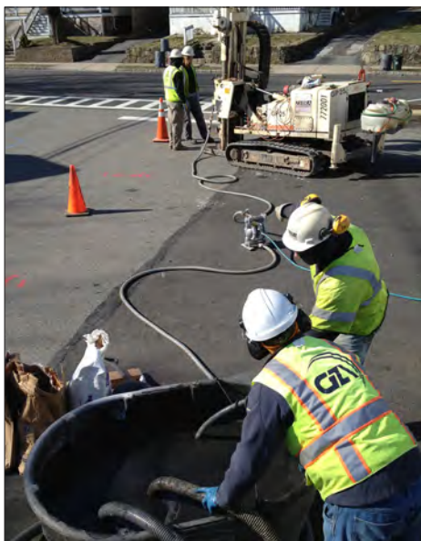
GZA personnel utilize in-situ biogeochemical remediation technologies
