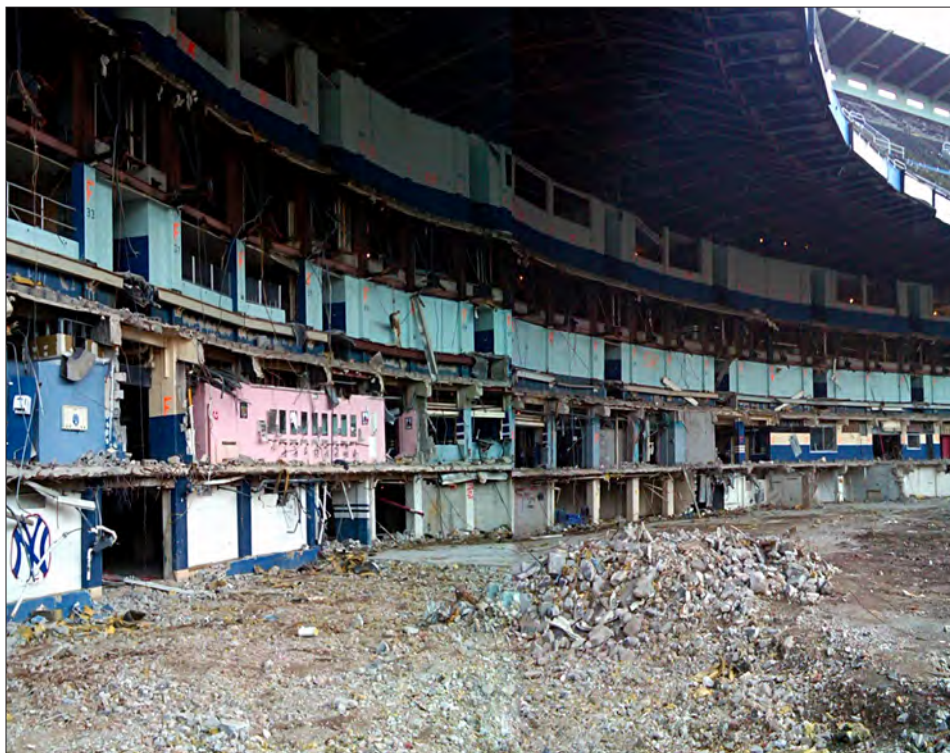
Hazardous materials and demolition assessments
