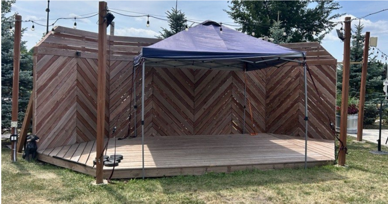
Existing stage to be demolished (above)
