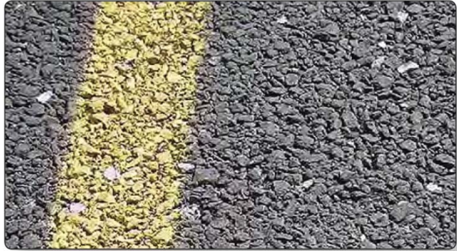
Figure 10-3. Example of Porous Pavement
