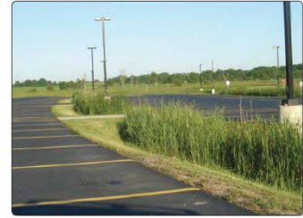
Figure 10-1. Example of Bioswales for Water Filtration.
