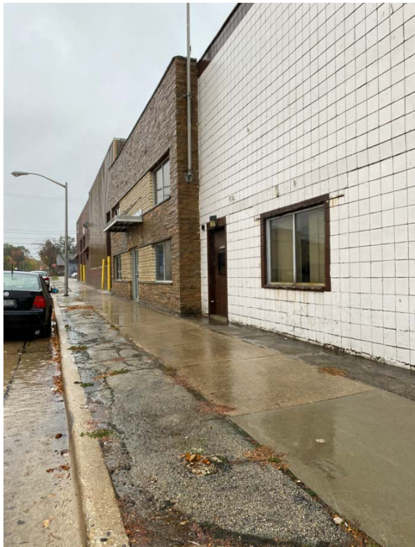
Above - Along S. 54 St. existing asphalt terrace conditions
