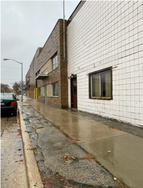
Above - Along S. 54 St. existing asphalt terrace conditions
