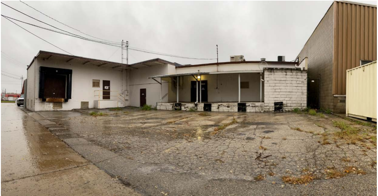
Above is the view from the alley (rear of building).
