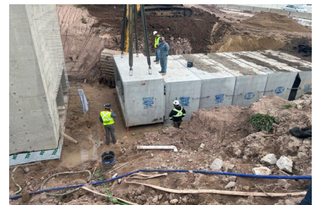
Fish creek box culvert
