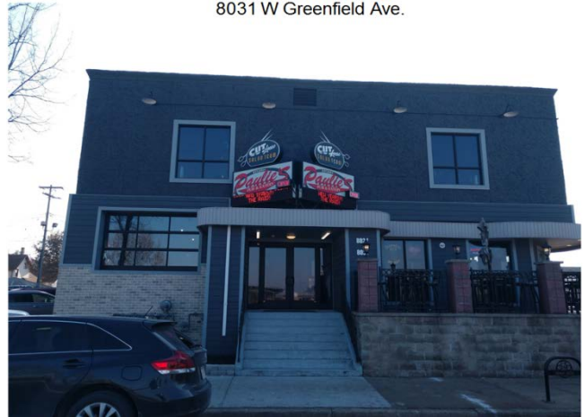
After Remodel (As built) – front entrance/north elevation 8031 W Greenfield Ave.
