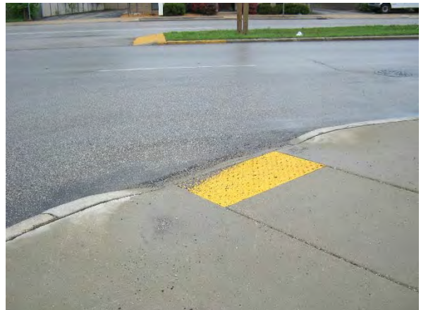
Curb ramp at National Avenue
