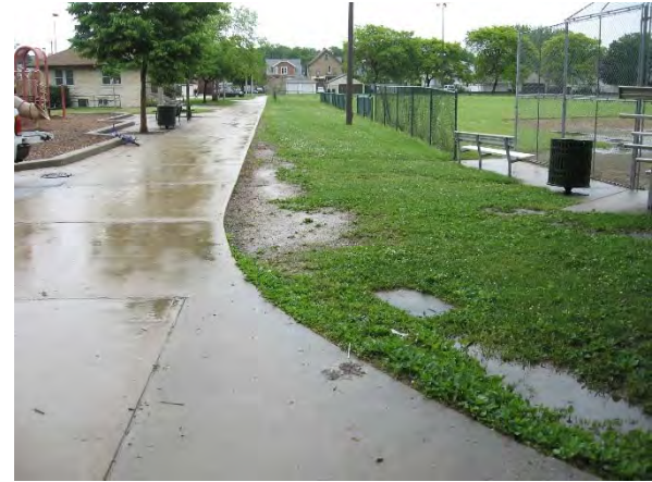
Erosion along path
