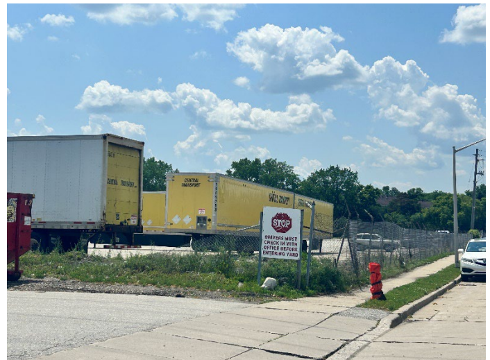
Fencing in disrepair and weed overgrowth
