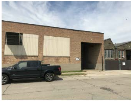
EXISTING CONDITIONS - PHOTO 11
