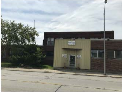
EXISTING CONDITIONS - PHOTO 2
