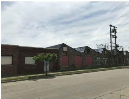
EXISTING CONDITIONS - PHOTO 6
