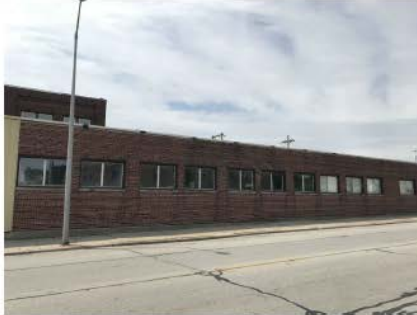
EXISTING CONDITIONS - PHOTO 3
