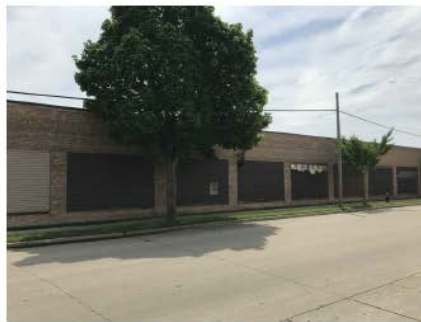
EXISTING CONDITIONS - PHOTO 7
