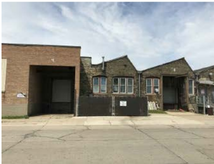
EXISTING CONDITIONS - PHOTO 10
