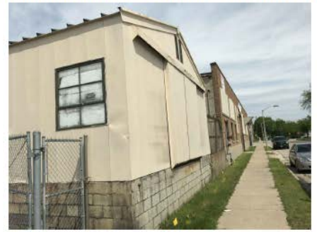
EXISTING CONDITIONS - PHOTO 12
