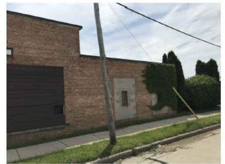
EXISTING CONDITIONS - PHOTO 8
