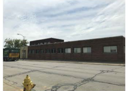
EXISTING CONDITIONS - PHOTO 4
