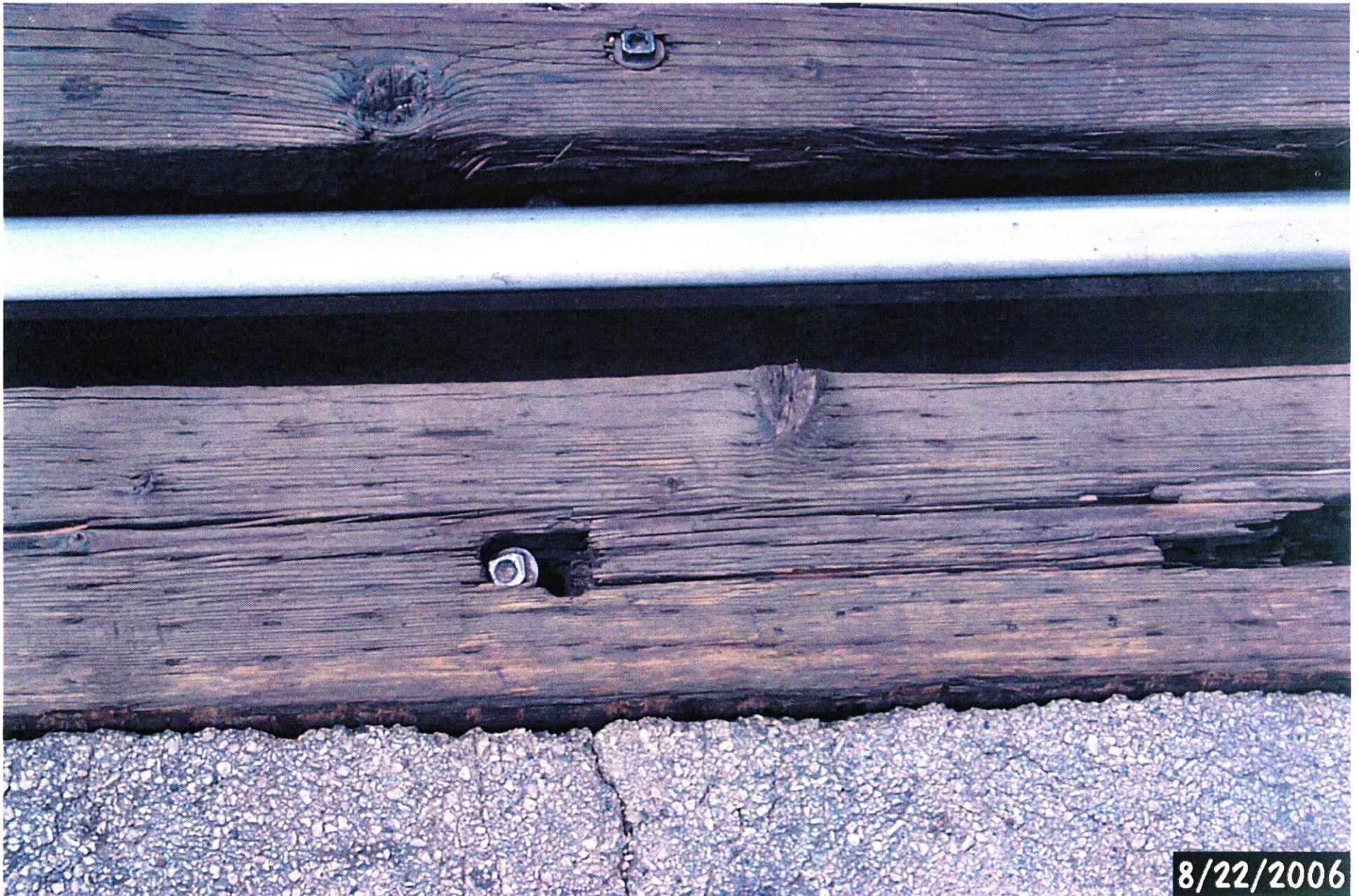
Picture taken by Brian Block on 08-22-06 of the Union Pacific at grade crossing in S 55 St-north tracks, rotted wood that rocks upward when traffic drives over.
