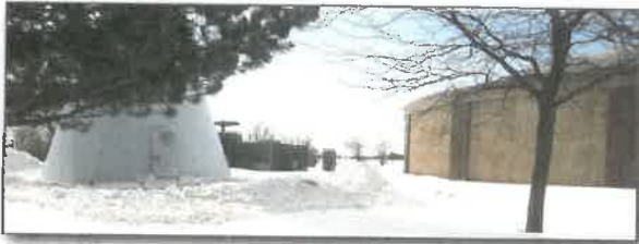
New generator addition location between reservoir and cell carrier compound.
