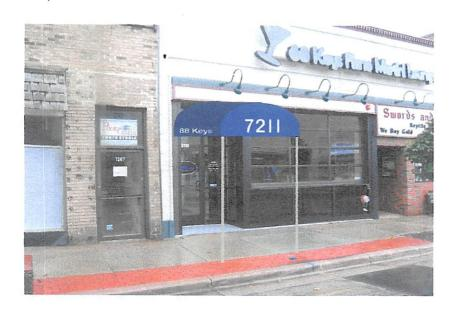
new awning, pac blue sunbrella 1" sq galv. welded frame, 6' wide 8'2" out, 3'0" high, 7'6" off ground 2" sq supports with 4" plate bottom at bottom( 4 holes with 3" anchors)
