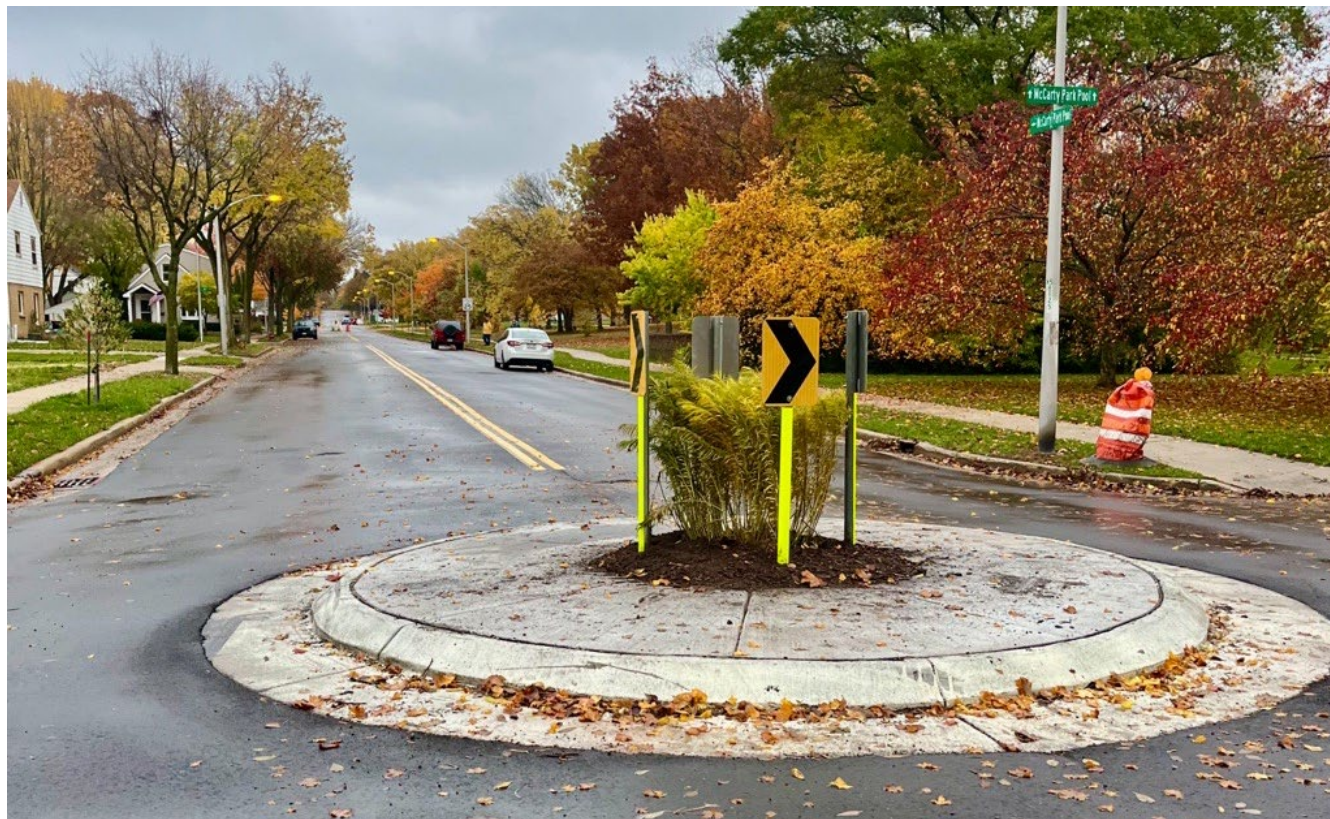
Traffic calming, like this traffic circle at 82nd & Arthur, create slower and safer streets for all users
