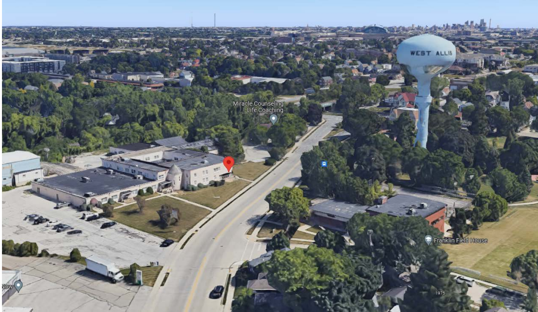
Existing bird's eye view of area – link to street view
