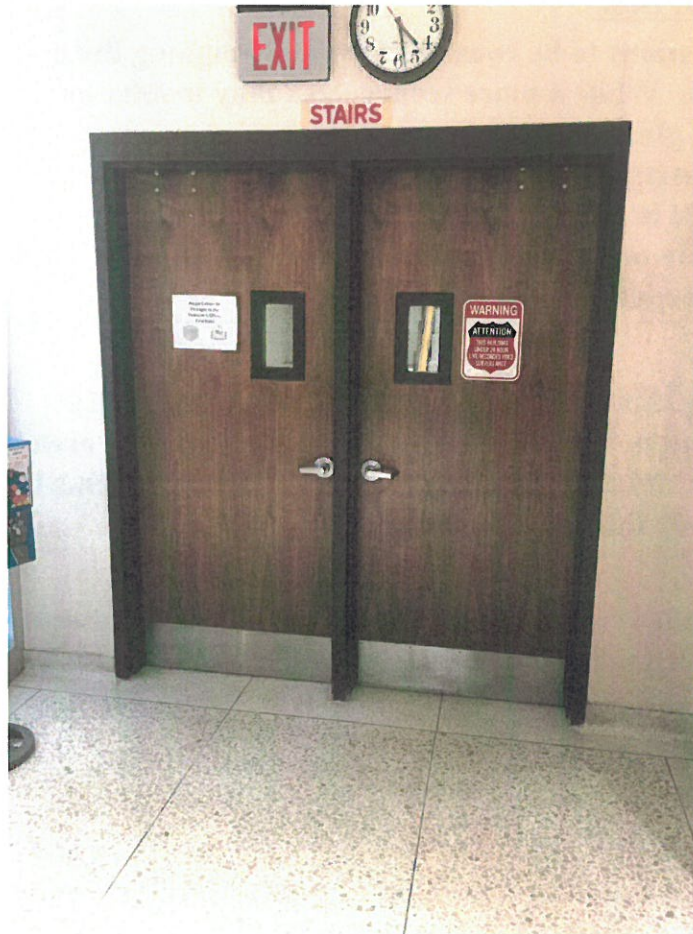
(Stairwell on Main Level of City Hall)
