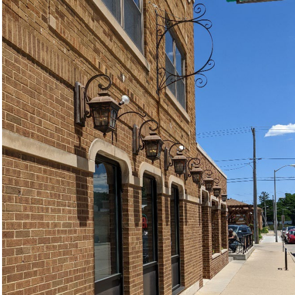
iii. Retaining historic features like the lights and original sign frame lend a historic feel to this building.
