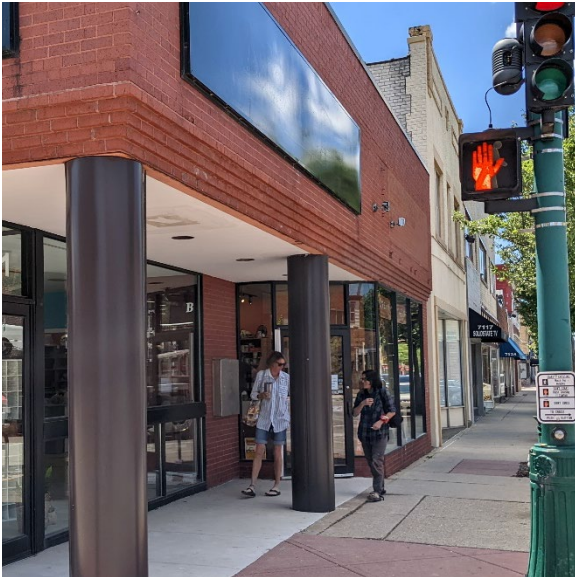
iii. Carving out building edges for a covered entry smooths the transition between the public and private realm, expands the sidewalk, provides weather protection and space for patrons to collect themselves.
