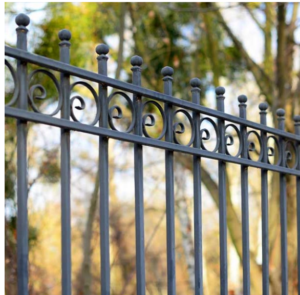
iv. Ornamental metal fencing delineates spaces in an attractive manner and adds character to a place, which is particularly beneficial along street frontages.
