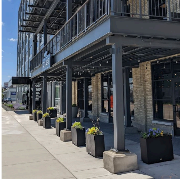
iv. This balcony addition references the historic industrial feel of the building while playing on the complementary colors of a neighboring building.
