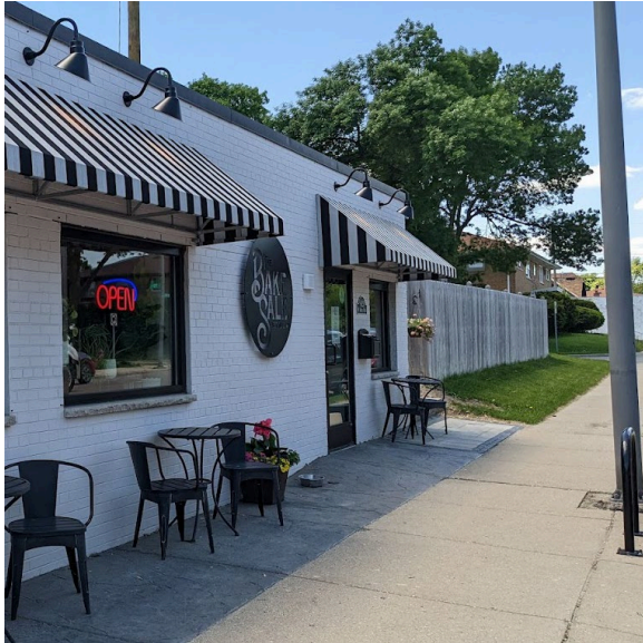
i. Orienting towards the street frontage enables an active streetscape and sense of place.
