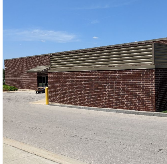
ii. Screening refuse containers within an alcove designed in concert with the materials of the building minimizes its impact.
